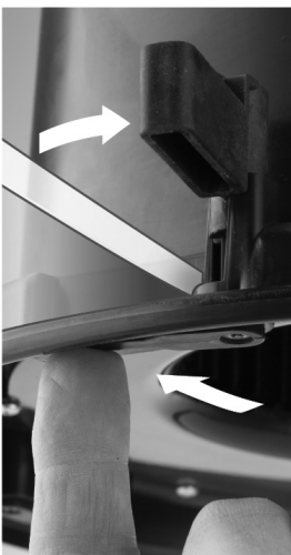
Rotate swing clips to hold fan body in place.
